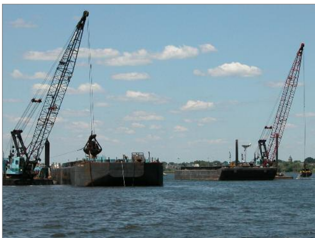
Donjon dredge's Newark Bay and Michigan loading the Dump Scow Witte 4001 and Hopper Scow Witte 3001 .
